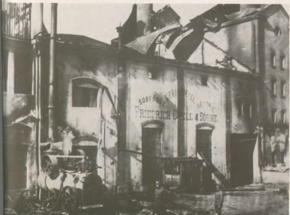
115. Brewery near Brassó damaged by shell-fire
