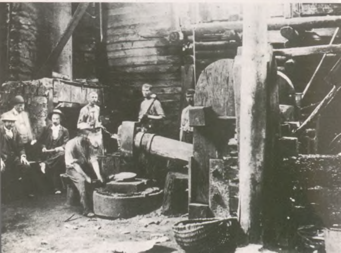
89. A medium-sized industrial concern: interior of the Lántzky foundry at Szentkeresztbánya at the beginning of the century
