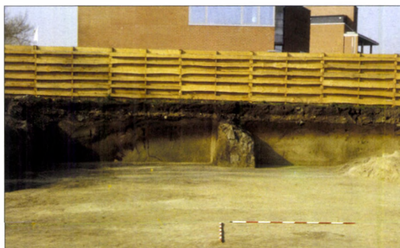
Picture 45. The line of the river bank with a steep Eastward inclination is clearly visible in the Southern profile of the foundation ditch of the modern building "C" of Graphisoft Park, Óbuda)
