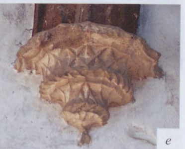
Fig. 150. a-e Corbels supporting a stellar vault, from the cloister walk of the northeastern palace
