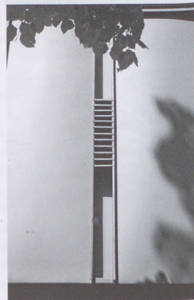
Fig. 50–51. The elevator built into a buttress of the chapel terrace, and a detail of its metal cover
