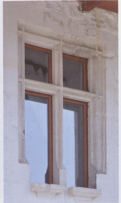
Fig. 161. Restored frame of a cross window from the ground floor of the western facade of the northeastern palace
