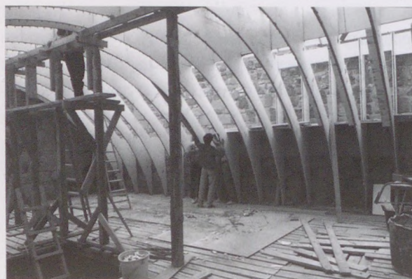
Fig. 34. The reconstruction of the southern wing. The gypsum concrete structure of the vaulted hall is prepared
