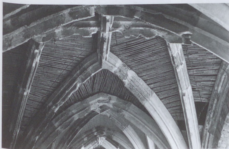
Fig. 230. Reconstruction of the cloister walk's vault, 1951
