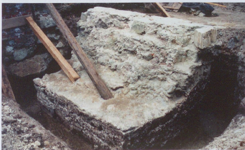
Fig. 36. A pillar foundation built of secondarily used carved stones, south of the southwestern corner of the northeast palace
