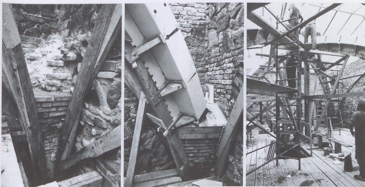
Fig. 53–55 Construction phases of the gypsum concrete structure in the cross vaulted hall on the upper floor, and how it adjoins the preserved remains of the vault
