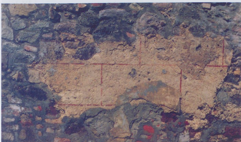
Fig. 90. Masonry lines painted in red on the external side of the palace's southern fence wall
