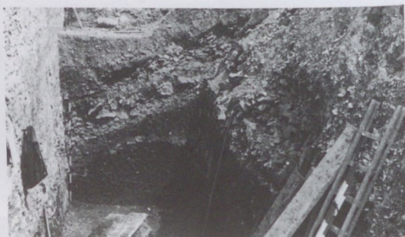
Fig. 226. Excavation of an embankment behind the retaining wall of the chapel terrace, 1959
