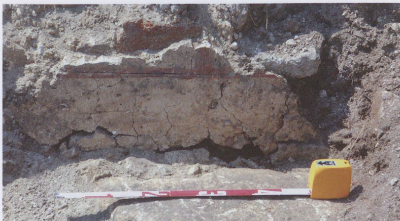
Fig. 89. Masonry lines painted in red on the building attached to the southern fence wall of the palace
