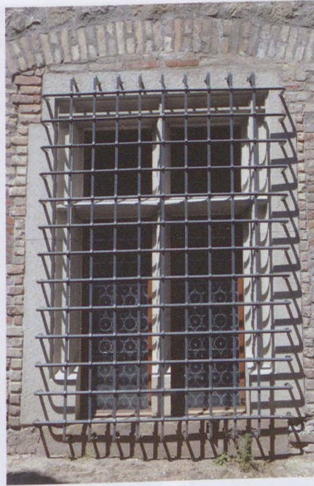
Fig. 160. Reconstruction of a frame of a cross window with iron bars from the eastern facade of the northeastern palace
