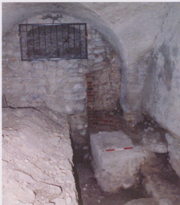
Fig. 32. The southeastern corner of the northern wing of the northeastern palace, with the springer of the arch leading to the western wing, as well as the foundation of the vaulting pillar
