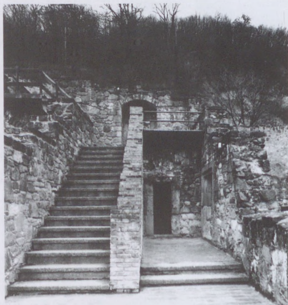
Fig. 12. The reconstructed lower part of the flight of stairs that led up from the loggia's level. The missing upper part was substituted with a concrete construction in order to make the Fountain of the Lions accessible
