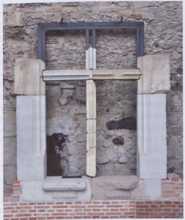
Fig. 163. Frame of a cross window from the northeastern palace
