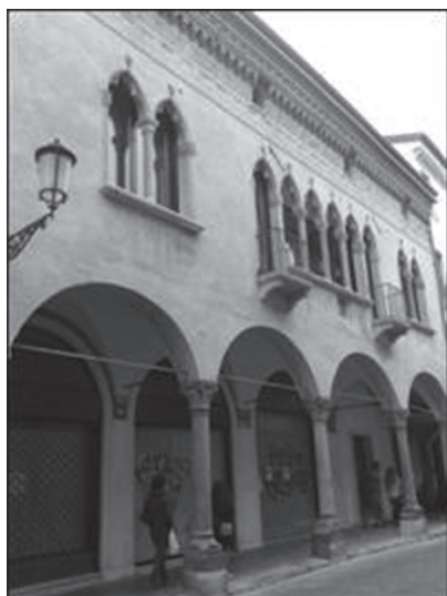
Fig. 9. The Pinelli House in Padua (known as Casa Casale, Via del Santo 127-131)
