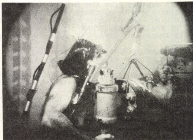
Fig. 1. Diver Breathing Helium-Oxygen Mixture While Performing Practical Work in Water-Filled Chamber at Pressure Equivalent to 488 Meters (1600 Feet of Sea Water) (8).
