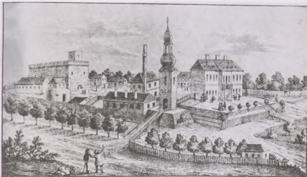
Ill. 5. View of the castle-building, the Ottoman cami , the Harruckern palace and the gate-tower, 1745
