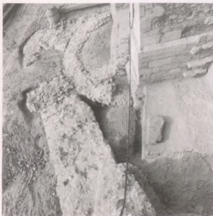
Ill. 8. Turkish defence work and its precursor in the Western Zwinger during the excavation. (Photograph by Margit Bakos)
