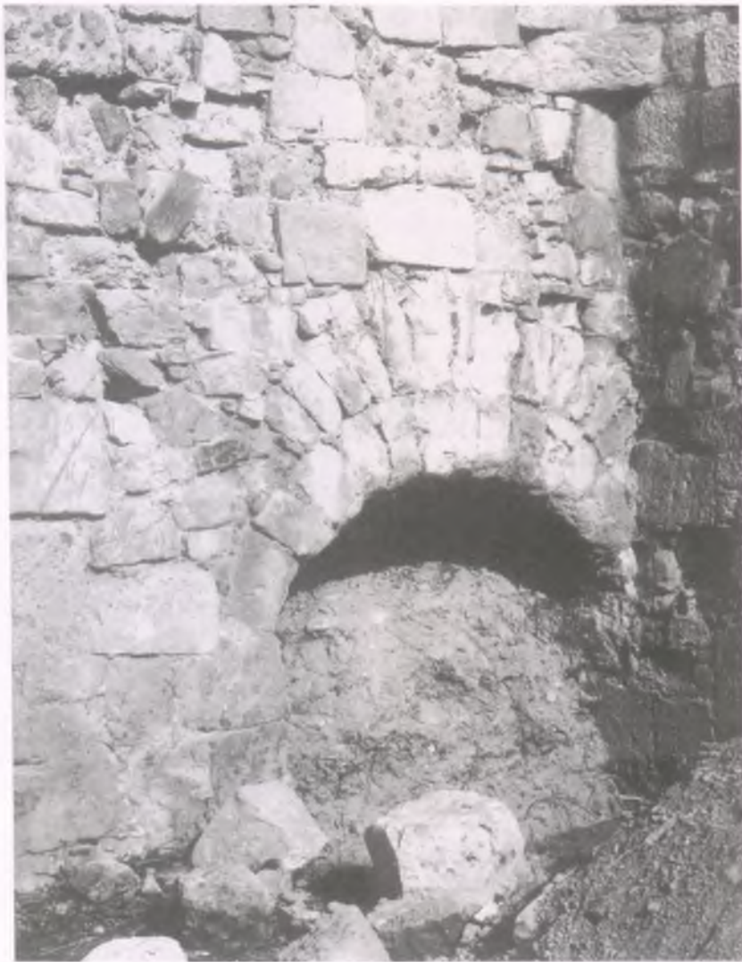
Ill. 7. The cleared Turkish gate leading from the Water-Town to the "Buda Gate" Round Bastion
