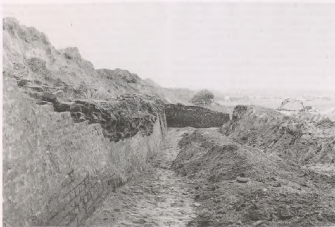
Ill. 3. Bajcsa-Vár. Brick buttress on the northern side. (Photograph: Ildikó Mazúr)
