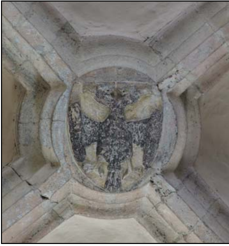
Fig. 3. Key stone from the central nave of the Cathedral of Alba Iulia displaying the arms of the Szécsi family
