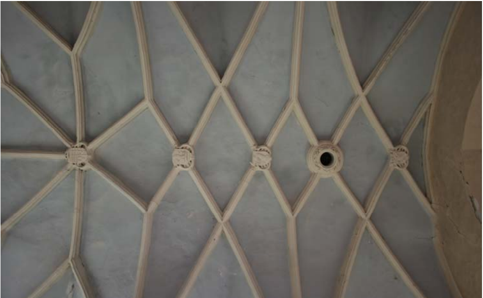
Fig. 12. The vaulting of the choir in the Vingard (Vingárd) church
