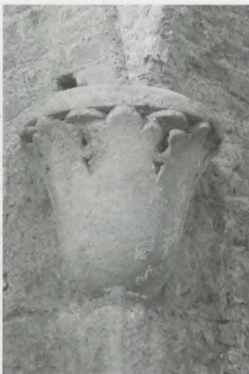
3. Corbel of the nave of the Abbey Church of Pilis, in secondary use in Esztergom, cellar of the Primate (Photo: Attila Mudrák, 2007)
