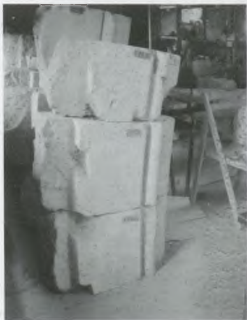
6. Vault ribs from the Abbey Church of Pilis, with holes in the side for inserting a support structure (Photo: Author)
