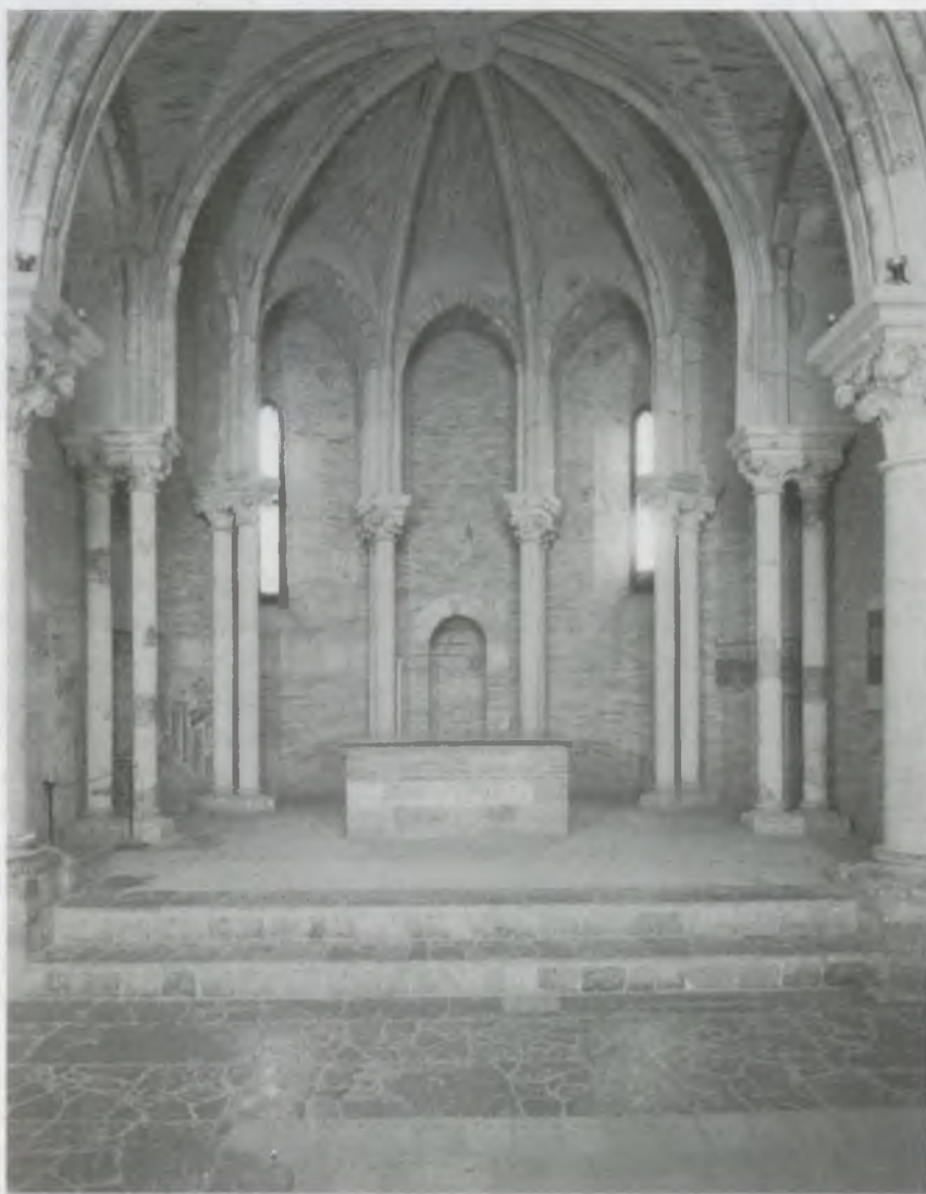
5. Choir of the Palace Chapel of Esztergom, reconstructed by Kálmán Lux in 1934–1938 (Photo: Róbert Hack, 1992, Photo Archives of the National Office for the Protection of Cultural Heritage, Budapest)
