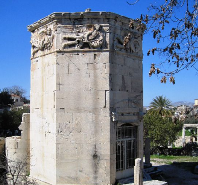
Figure 2: Tower of the Winds clocktower in Athens, Greece. The tower had 9 sundials on the walls and a water clock inside driven by water flow from the Acropolis. (Photo: Herczeg, T.)
