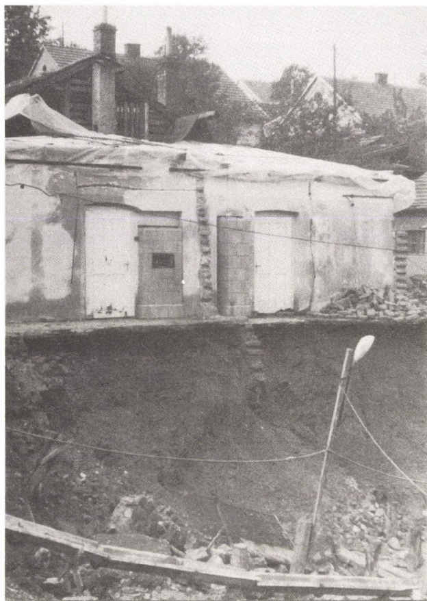
Picture 3. Landslip and damage due to building disruption: Komló
