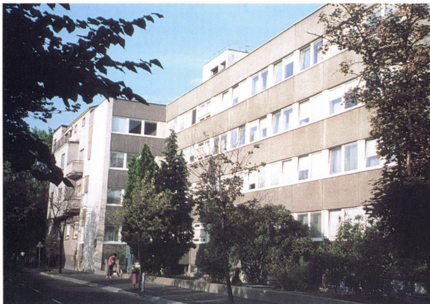
The main building of the Institute
