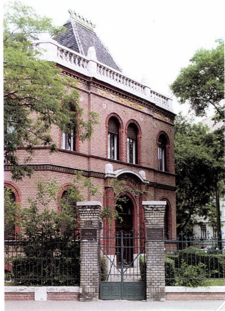
The main building of the Institute
