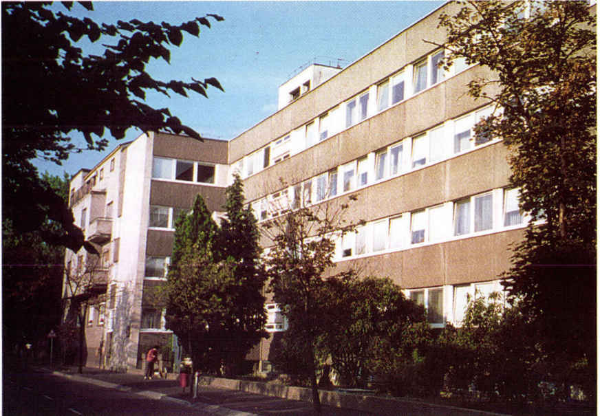
The main building of the Institute
