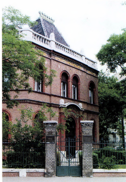
The main building of the Institute
