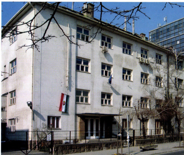
The main building of the institute
