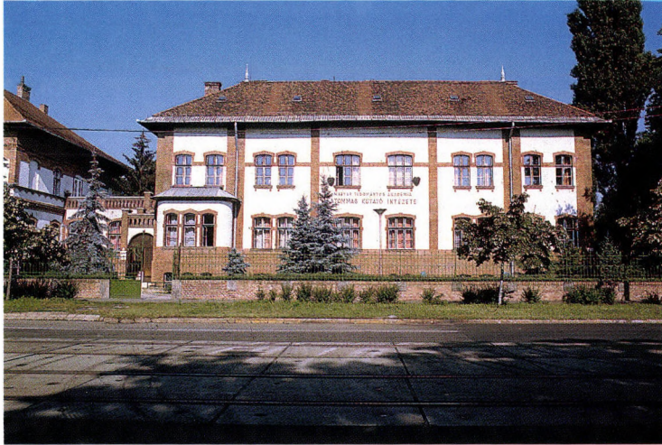
The main building of the institute
