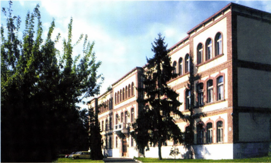
View of the main building of the research institute
