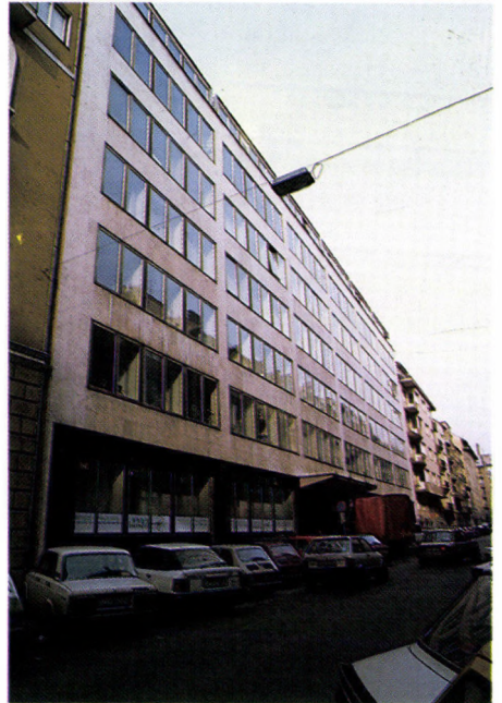
The main building of the institute
