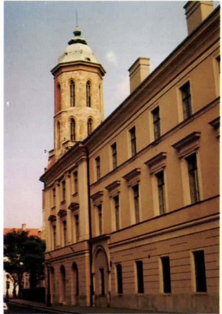
The main building of the institute
