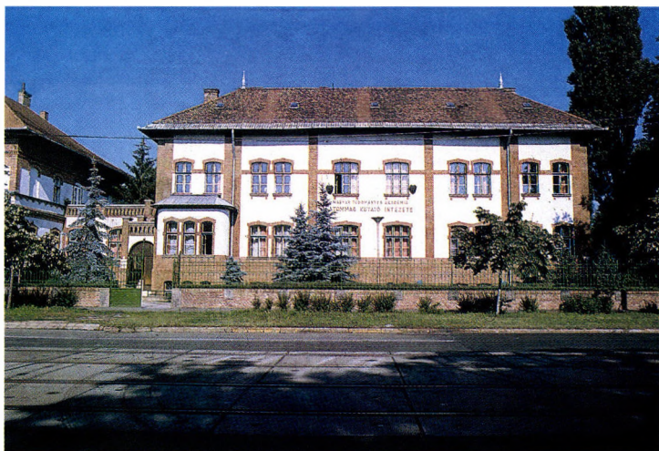
The main building of the institute
