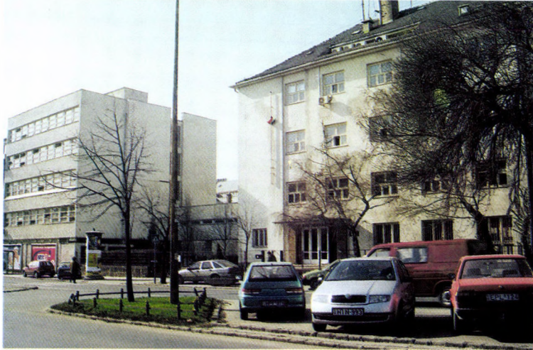
The main building of the institute
