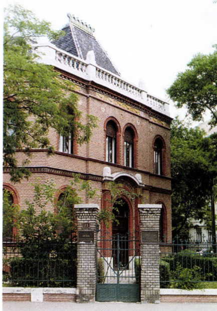
The main building of the Institute
