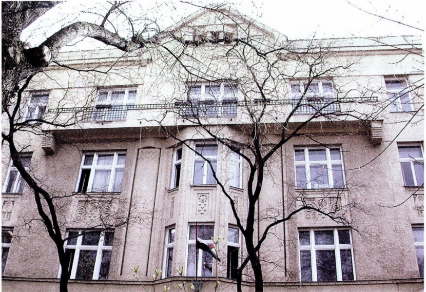
The main building of the institute
