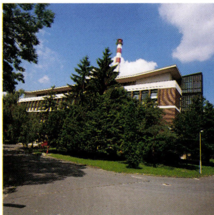
The main building of the research Reactor
