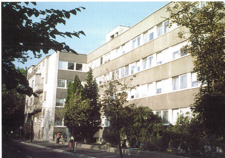
The main building of the Institute
