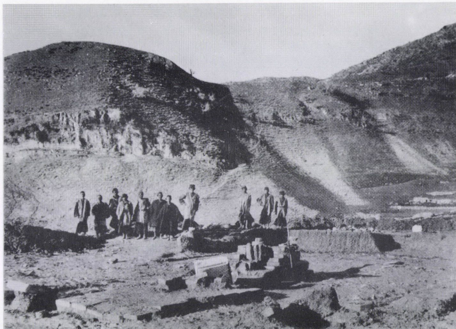
52. REMAINS OF SHAMĪ SHRINE, SEEN FROM NORTH-EAST
