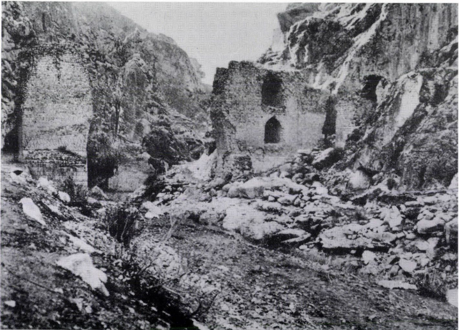
83. RUINED BRIDGE ACROSS KĀSHGĀN RIVER AT KALHŪR, PĪSH-I-KŌH
