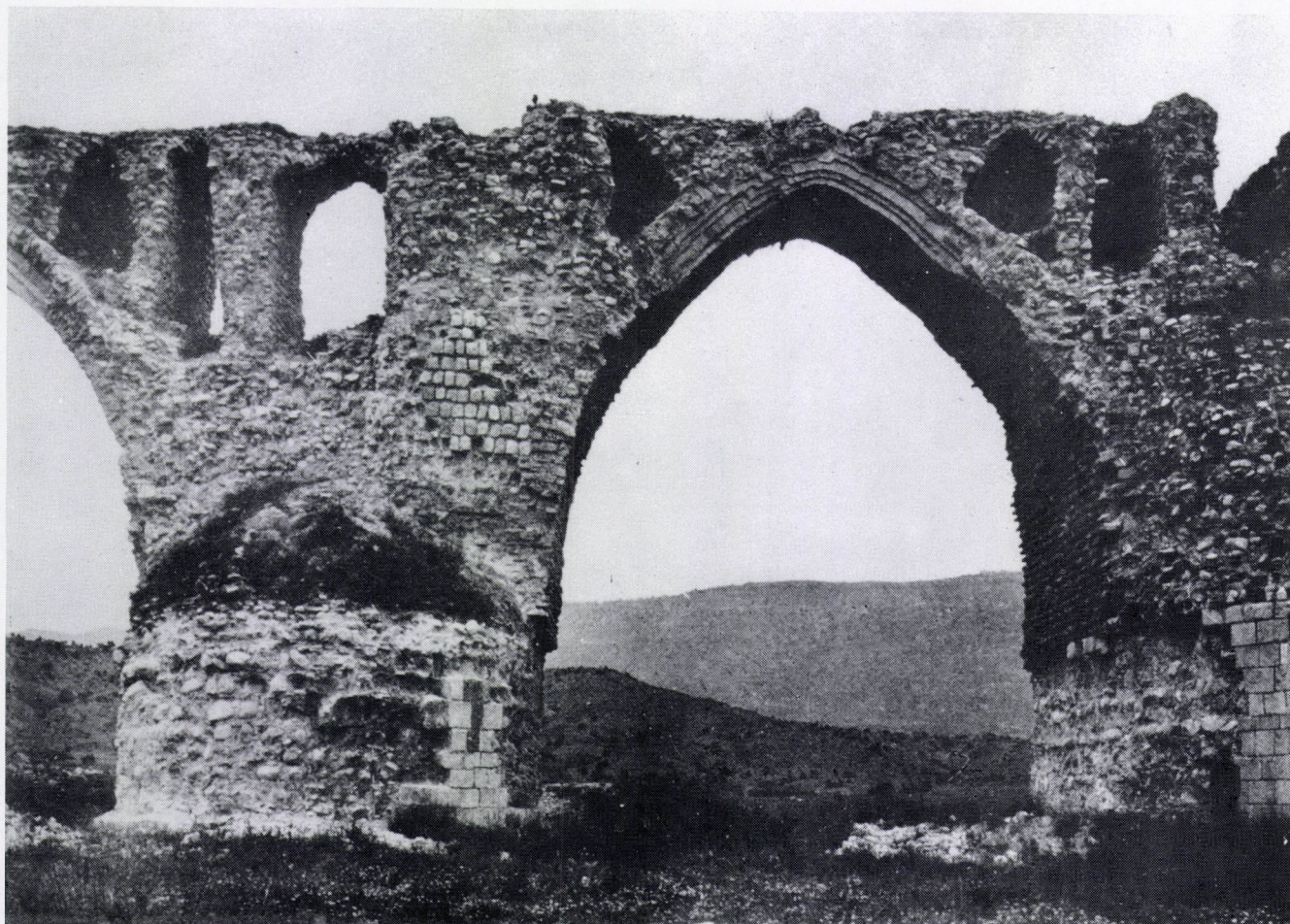
SI. ARCH BETWEEN PIERS V AND VI, PUL-I-KĀSHGĀN, SUMĀQ
