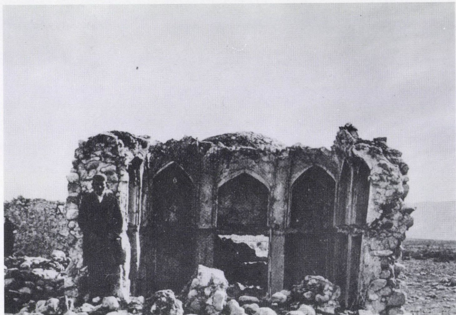
26. INTERIOR OF RUINED HOUSE AT AULISH, TĀSHĀN
