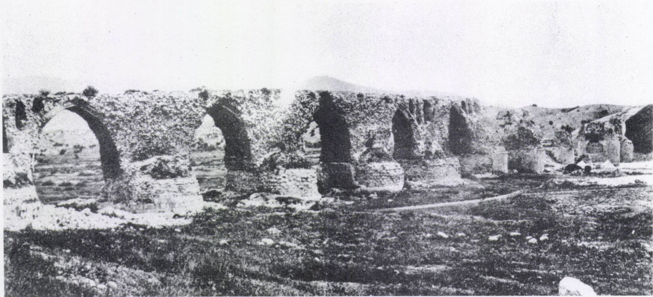
80. RUINED BRIDGE ACROSS KĀSHIGĀN RIVER, SUMĀQ, SEEN FROM RIGHT BANK
