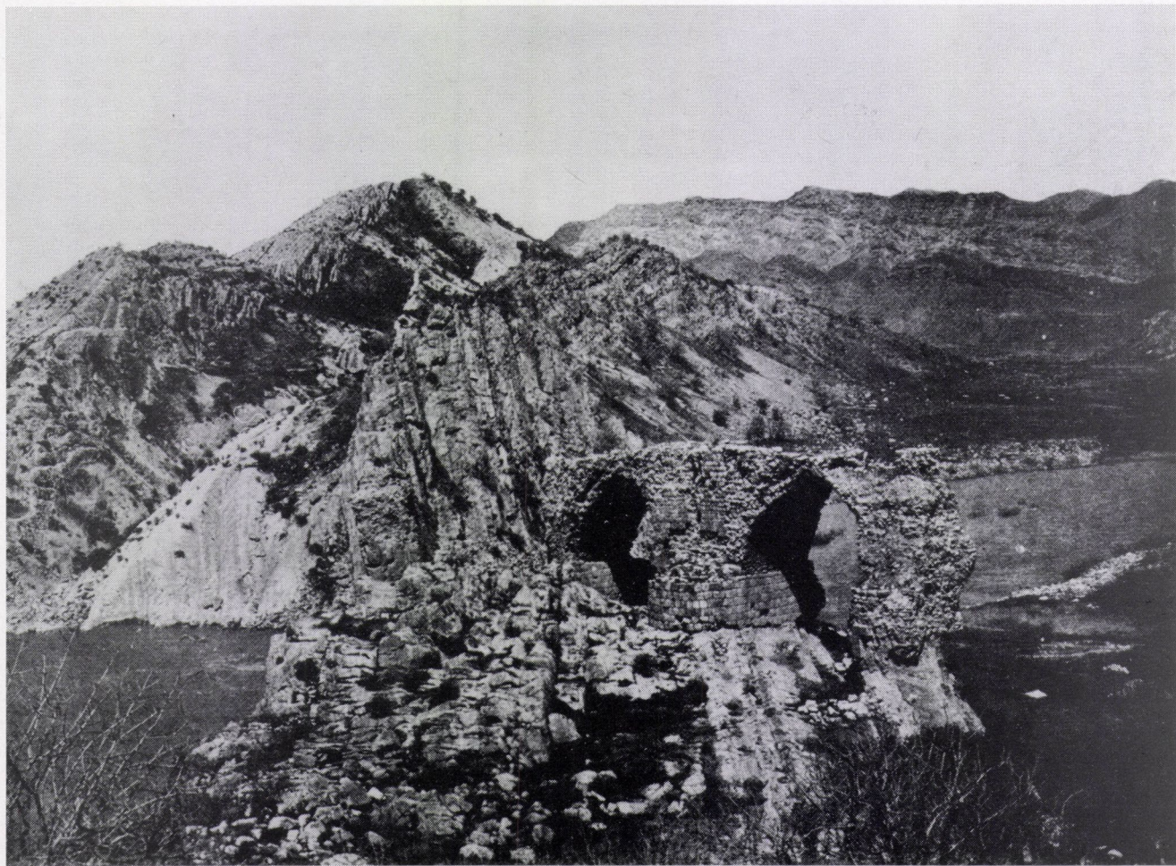
73. RUINED BRIDGE ACROSS SAIMAREH AT SEFALEH, HULAILĀN
