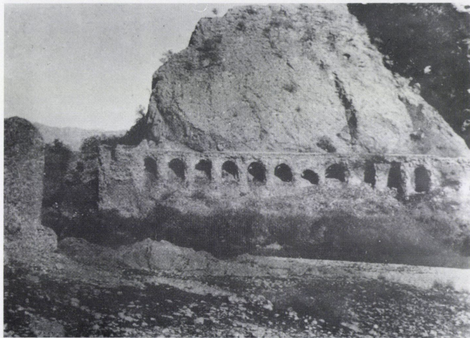
16. PUL-I-BRĪN, WITH ARCHES OF APPROACH ON LEFT BANK TO LOWER BRIDGE
