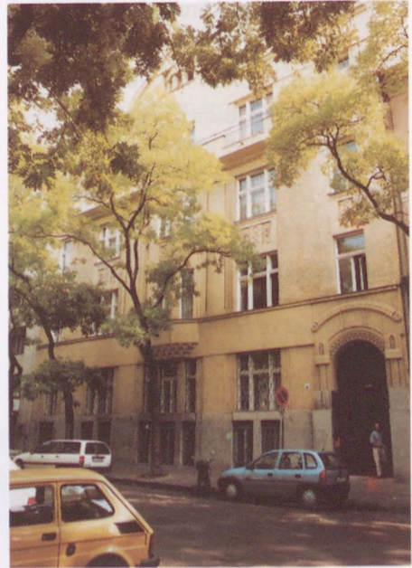
The research building which houses both the Institute for Political Sciences and the Institute for Social Conflict Research. (Photo Mérei)
