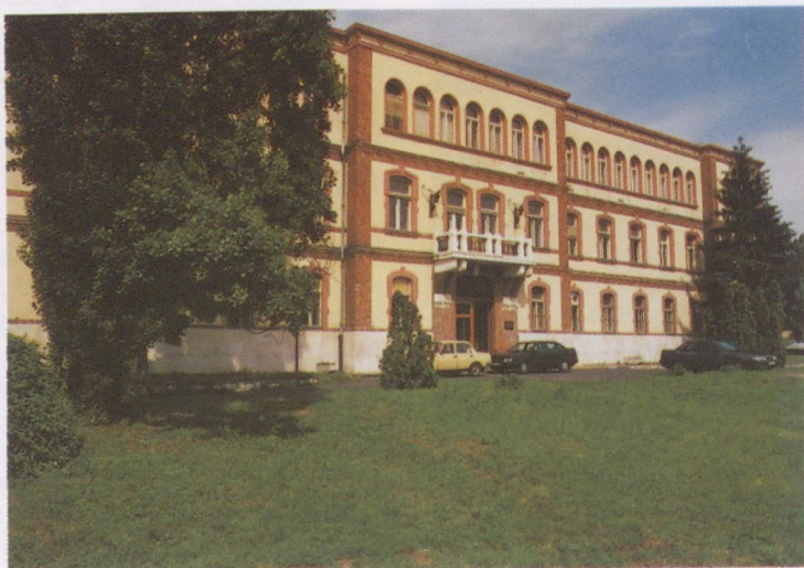
View of the main building of the research institute
