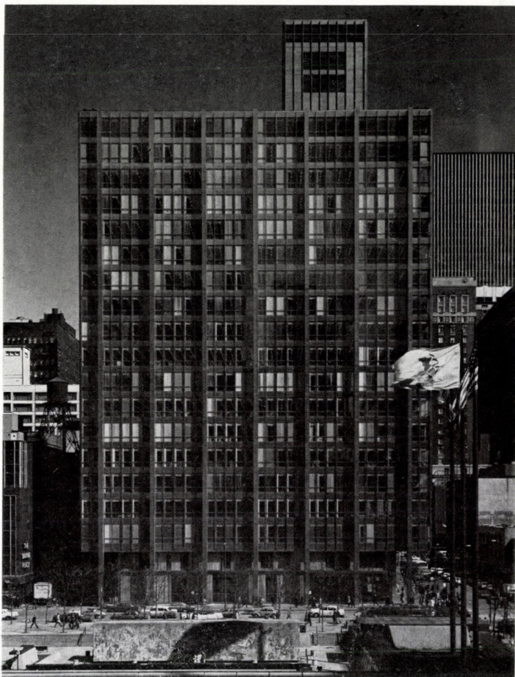
INLAND STEEL BUILDING, CHICAGO, ILLINOIS, 1958.
